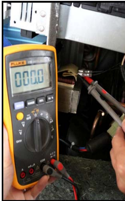
Fig. 33 – Test the Reactor Resistance
